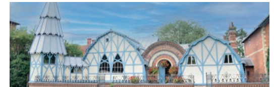
Pump Rooms, Tenbury Wells
